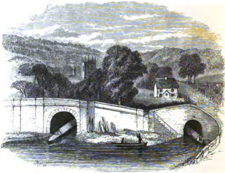
NORTHERN ENTRANCE OF HARECASTLE TUNNELS 1
